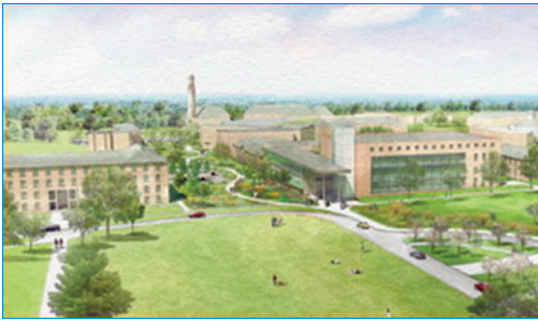
A new Interdisciplinary Computational Science Research Center (on right) is slated to be built on the north side of campus.
